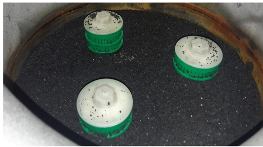
a) bottom nozzles, b) flow and air pressure control and connections for washwater and air
