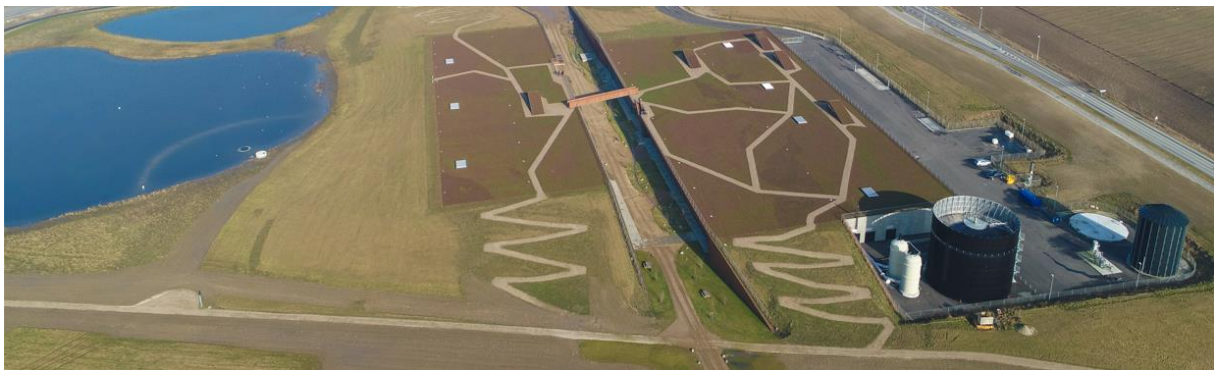
Figure 2. WWTP in Hillerød. The pretreatment, process tanks and clarifiers with pumps etc. are fully covered inside two buildings built in the landscape with green roofs.
