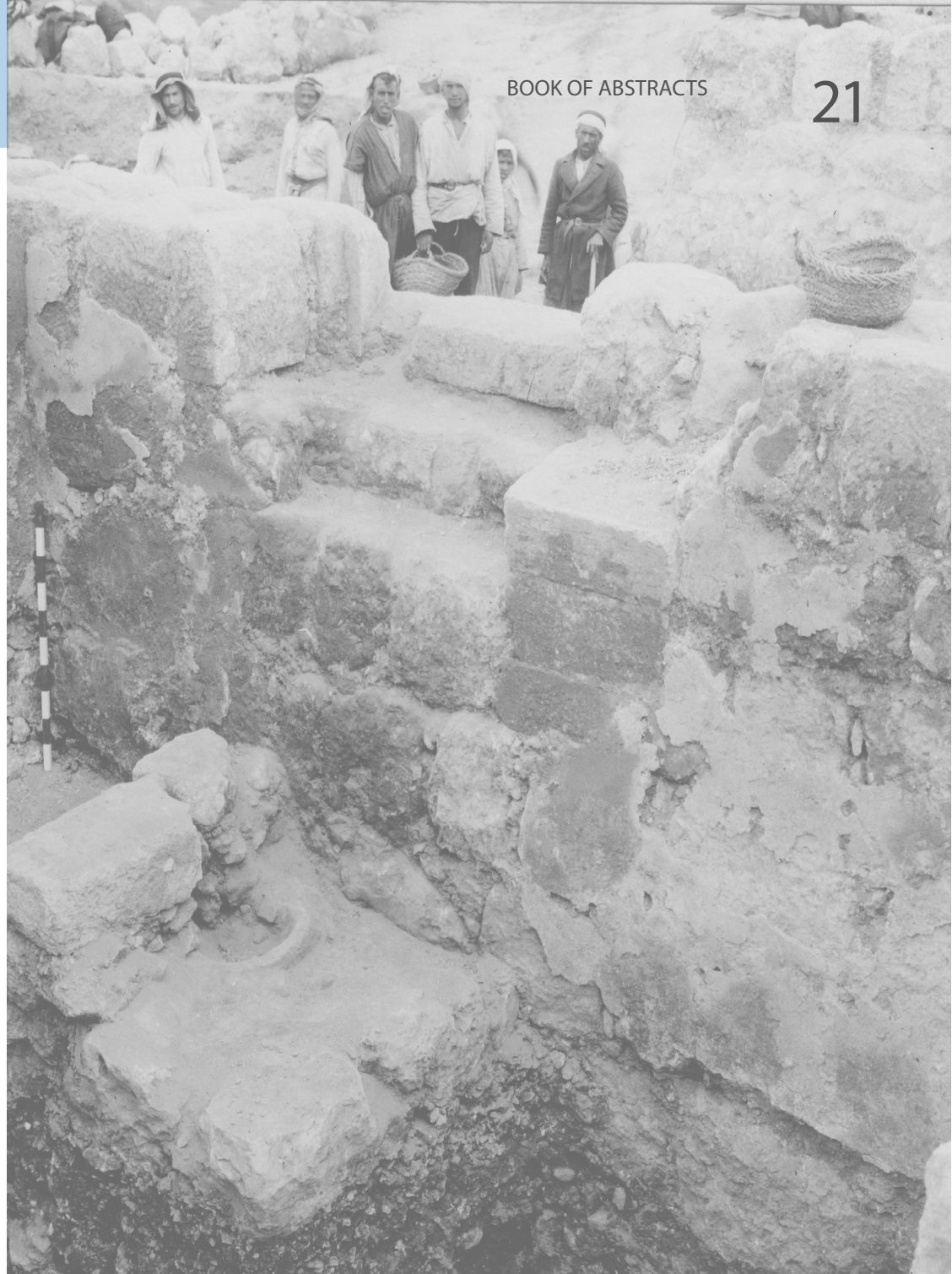
South-east of Camp Hill, Room 1 looking south-east with workers posing behind the wall (17 April 1931). Photos courtesy of Yale University Art Gallery.
