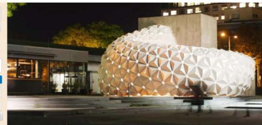
The ArtoSkin bioplastic facade created by Stuttgart University's ITKE (Institute of Building Construction and Structural Design) demonstrates the possible architectural and constructional applications of bioplastic materials. | Image credit: Institute for Building Construction and Structural Design
